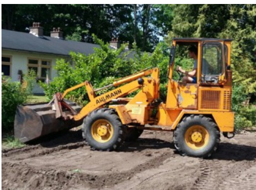
Wim levelling ground with the bulldozer
